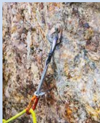
New, longer stainless steel bolts (left) are glued into the rock. They won't rust, unlike bolts put in decades ago (right), which are shorter. (Eric Barnard)
