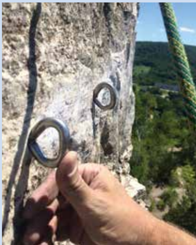
New, longer stainless steel bolts (left) are glued into the rock. They won't rust, unlike bolts put in decades ago (right), which are shorter. (Eric Barnard)
