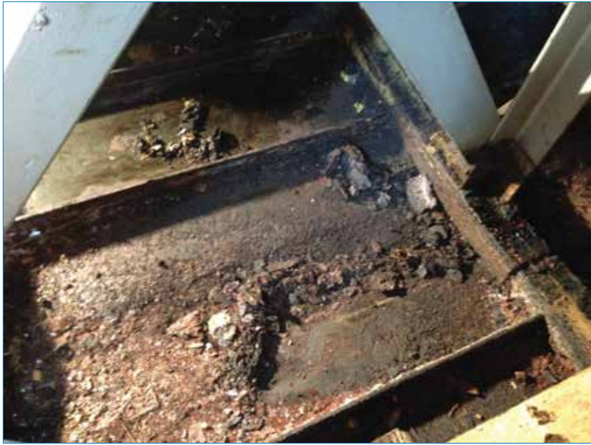
The inside of the hull was in bad shape (left) before it was cleaned and painted (right).
