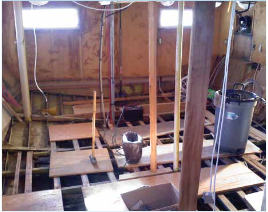
The interior walls, floors and ceilings had to be removed.
